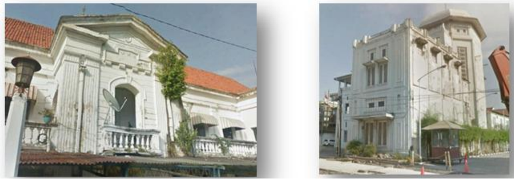
Figure 4: The facade of an ancient building today
